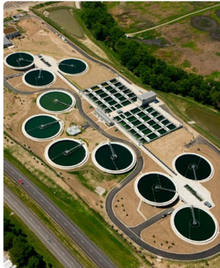
Aerial view of Spring Creek Wastewater Treatment Plant PHOTO: Courtesy of Terry Farmer Photography
